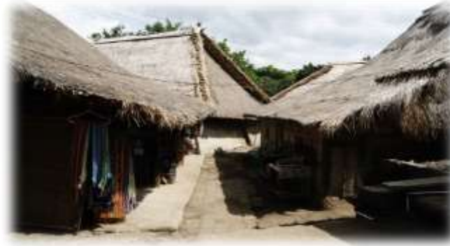
Figure 3. The Roof of the Bale Tani House
